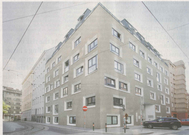
More than a shelter, built by WBV-GPA : At neunerhaus Hagenmüllergasse in Vienna 79 formerly homeless people receive privacy, autonomy and a home.
